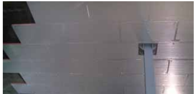
Figure 6 Board joints squared
